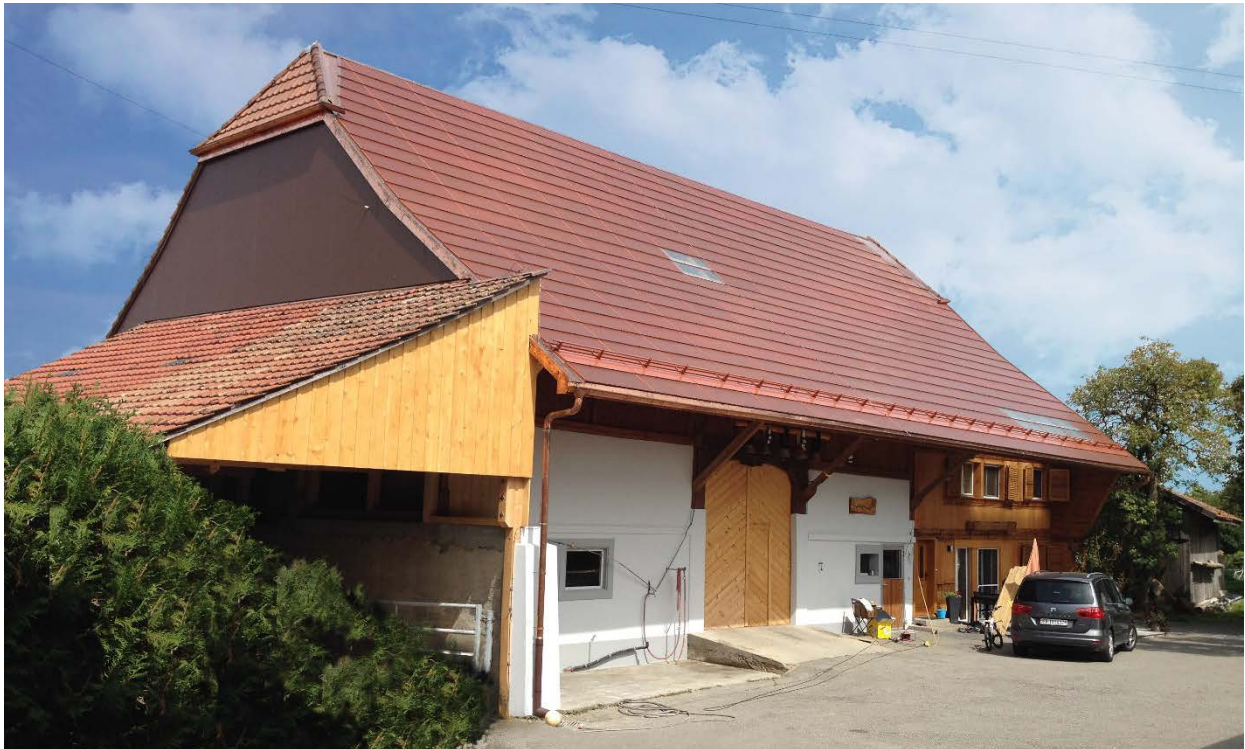
Perfect integration: terracotta-red solar panels, Ecuwillens/FR Switzerland pilot project
