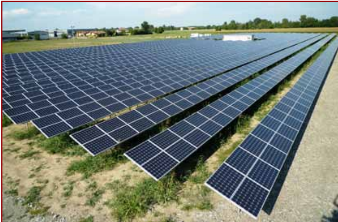
Fig. 1.1: Moduli policristallini posati in un impianto in Italia Fig. 1.1: Polycrystalline modules in an italian plant
