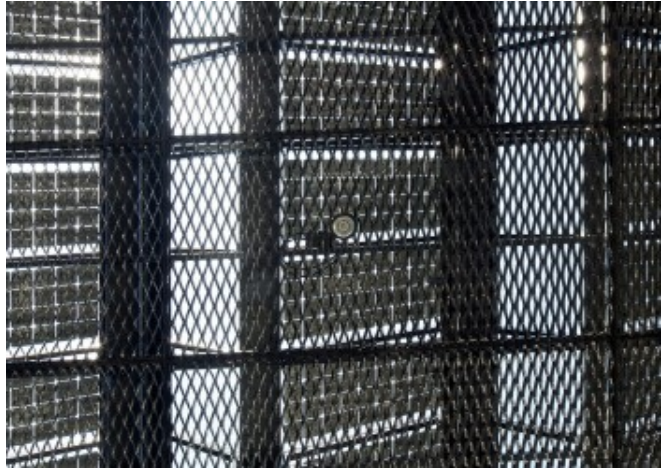
View of the glass photovoltaic roof and the black aluminium grill placed below © Günter Richard Wett
