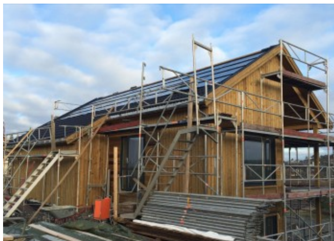
Building site after BIPV installation © Inger Andresen (ZEB Sintef/NTNU)
