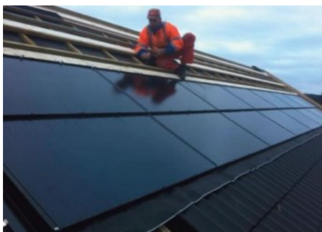
Mounting of the BIPV modules © Skanska
