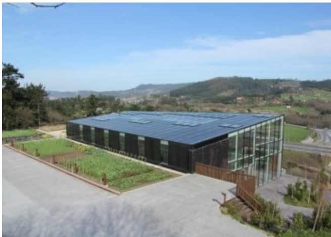
BIPV roof and façade of Azurmendi restaurant © Naia Eguino
