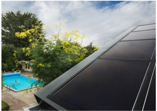
Design solution connection BIPV and eaves © Beausolar
