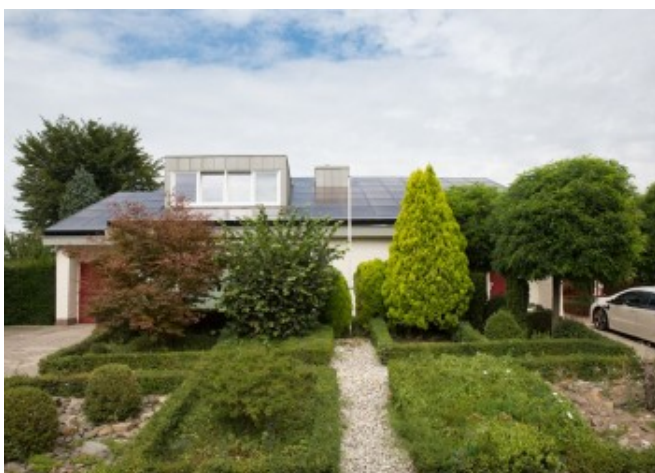
Street view showing the full roof BIPV © BEAU solar
