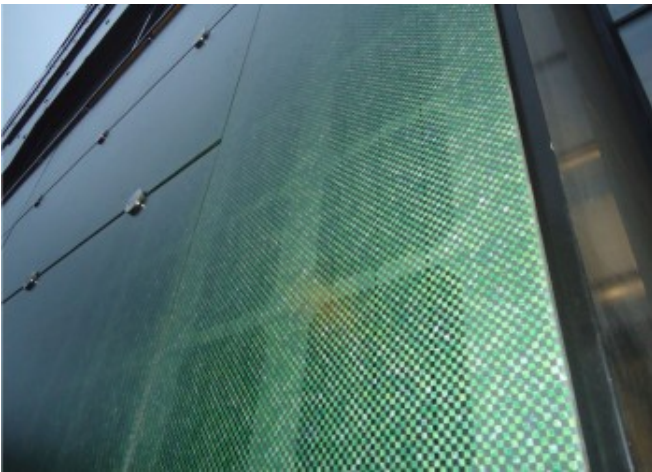
Detail of the green screen-printed module © Åse Lekang Sørensen (Norsk Solenergiforening)
