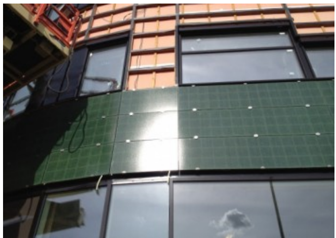
Mounting BIPV modules on a curved section © FUSen
