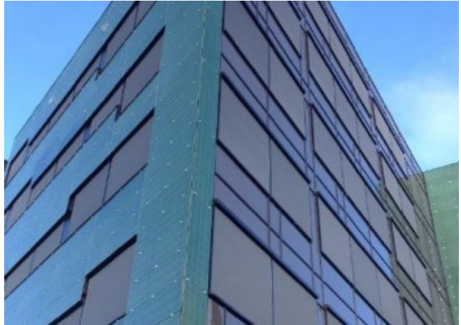
BIPV and glass façade © FUSen
