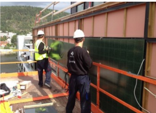
Mounting of the BIPV façade modules © FUSen
