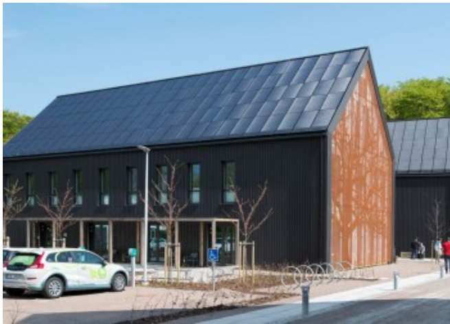
South façade and BIPV roof © Skanska Klas Andersson
