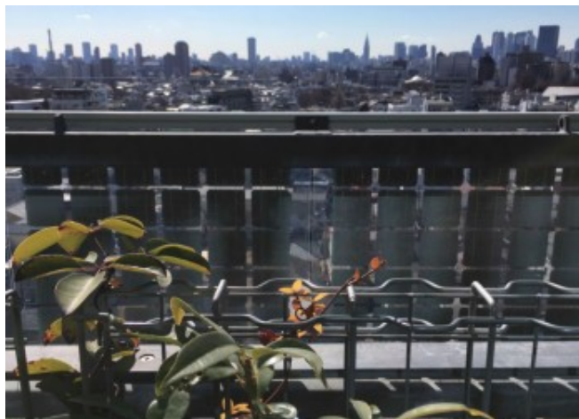
Inside view of the BIPV balustrades
