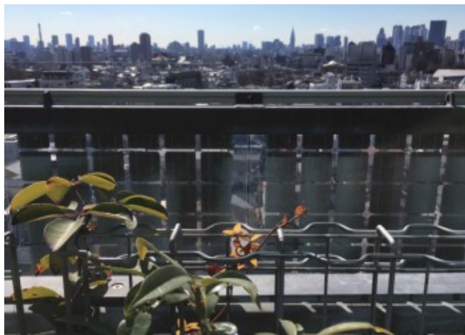
Inside view of the BIPV balustrades
