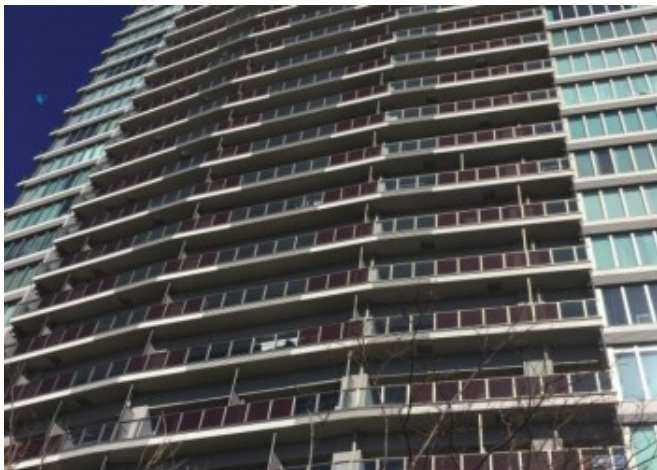
BIPV on residential façade
