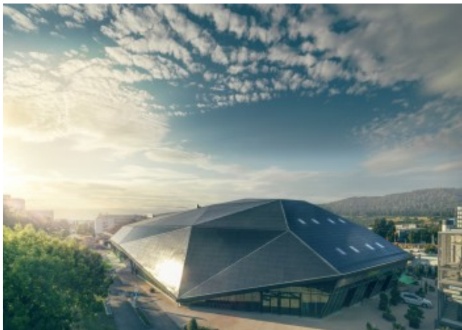
BIPV roof overview © René Schmid Architekten AG
