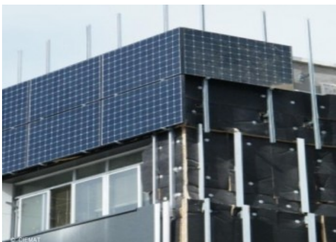
Renovation work details. PV modules mounting © CIEMAT
