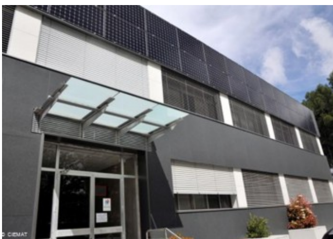
Renovation work finished © CIEMAT
