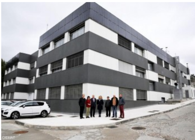
CIEMAT office with project team © CIEMAT
