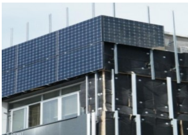
Renovation work details. PV modules mounting © CIEMAT
