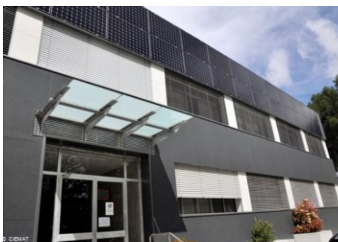
Renovation work finished © CIEMAT
