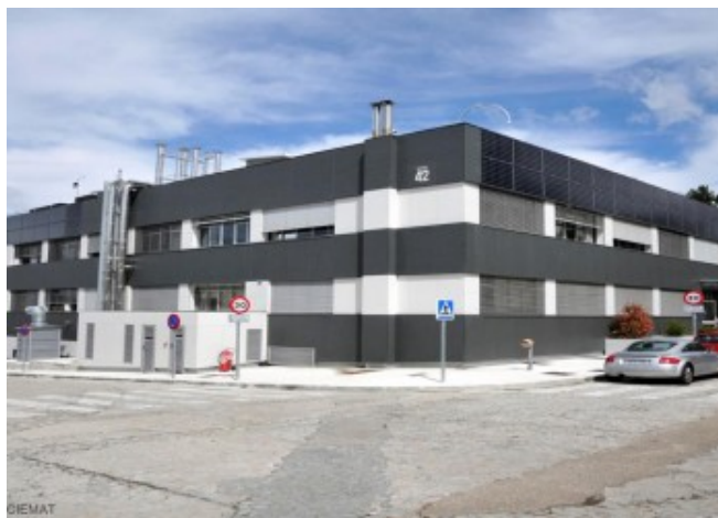
CIEMAT office with the access road © CIEMAT
