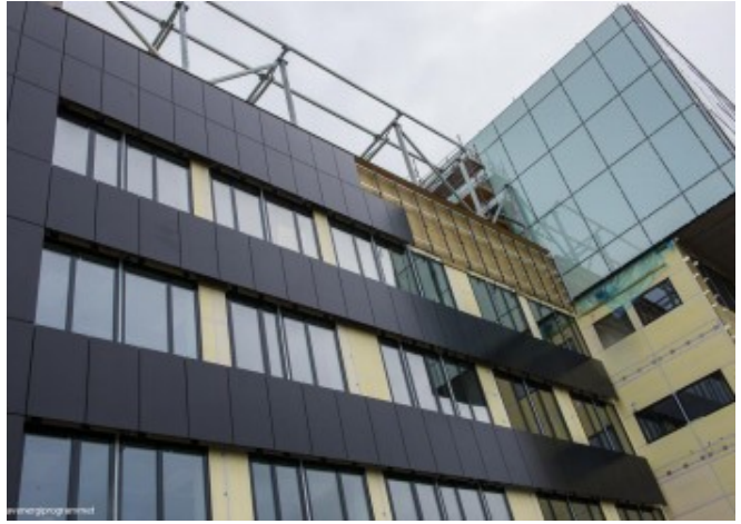
Mounting of the BIPV façade modules © Lavenergiprogrammet
