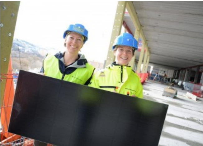
Environmental advisor and technical project manager © Undervisningsbygg Oslo KF
