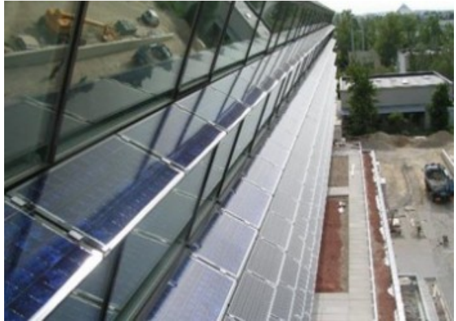
Folded BIPV façade © AIT-POS Architekten
