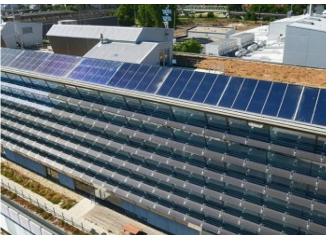
Zig-zag-BIPV façade with six stripes of PV and solar thermal collectors on the top © AIT-Johannes Zinner
