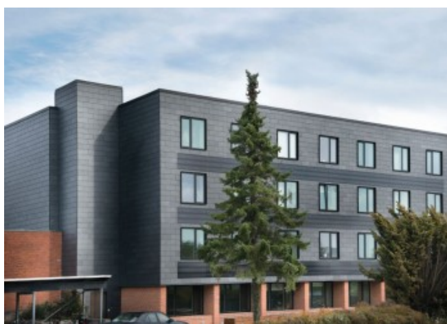
BIPV façade © KANT Architecter
