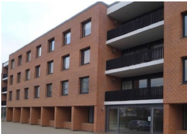
Apartments before the renovation © KANT Architecter
