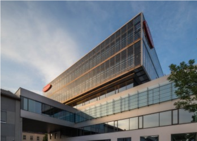
BIPV South-West façades © Dieter Moor, ertex solartechnik GmbH
