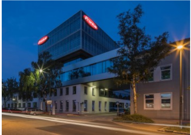
Dummy modules on the North façade © Dieter Moor, ertex solartechnik GmbH
