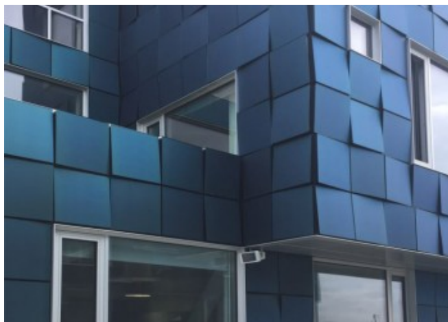
Detail of BIPV façade © Karin Kappel
