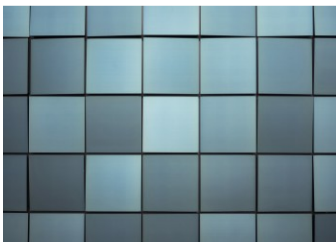
Close-up of the façade: the colours are depending on the angle of the module © C.F. Møller Architects / Adam Mørk
