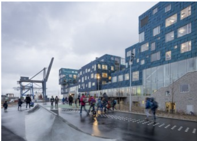
BIPV north façade © C.F. Møller Architects / Adam Mørk
