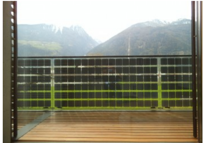
The semitransparent railing allows to enjoy the landscape from inside © building owner
