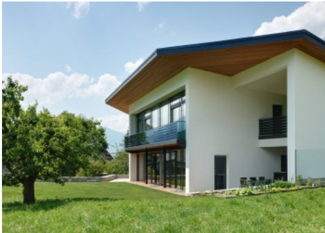
View of the two photovoltaic railings © building owner
