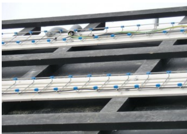
Wood modules substructure: the cables and the fire-resistant plasterboard are visible © Leitner Electro Srl
