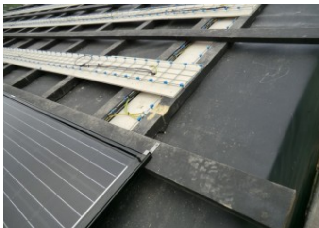
Detailed view of the 'Solrif' mounting system © Leitner Electro Srl
