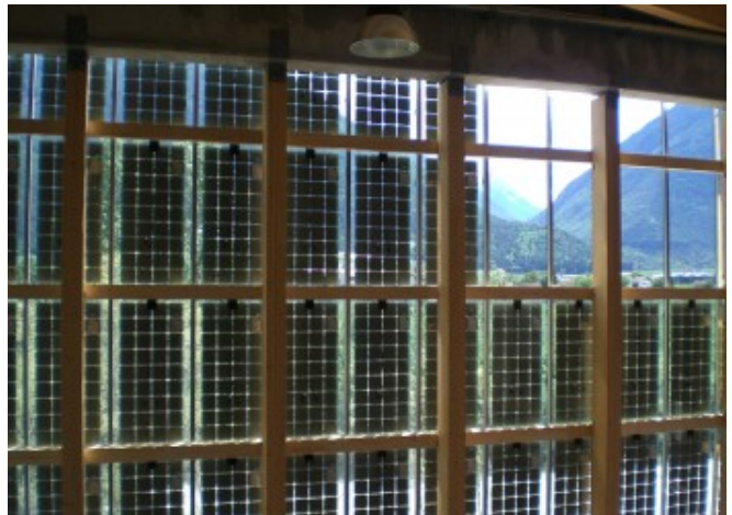
View from inside the building: the supporting wood structure and the modules semi-transparency are visible © Günther Wallnöfer
