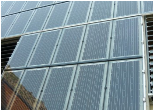
Detailed view of the semi-transparent frameless modules © Günther Wallnöfer
