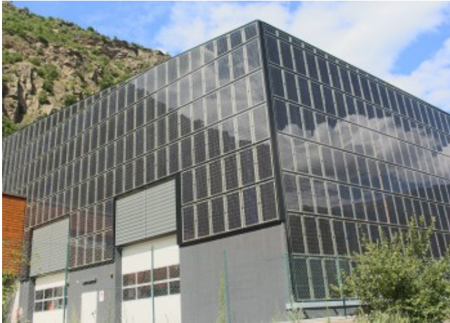
The plant covers the opaque parts as a cold façade system generating a stack effect © Eng. Klaus Fleischmann
