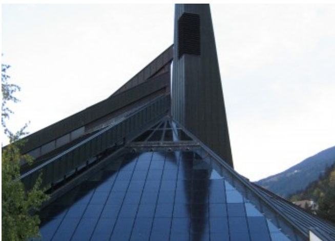
First fake modules installed, too reflective © Eurac Research
