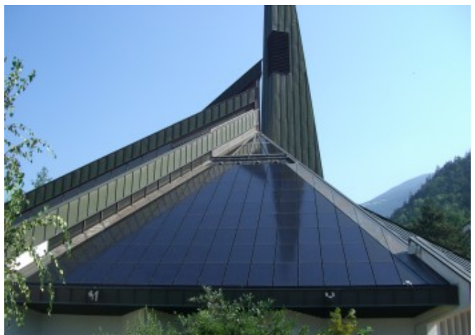
Final fake modules installed, matching the BIPV plant surface © Eurac Research
