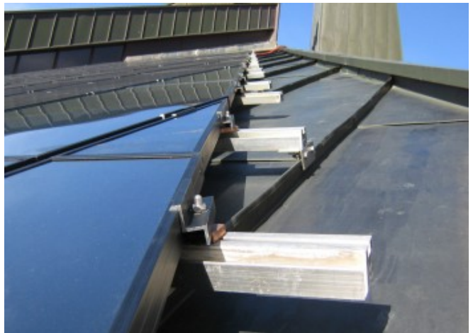
Detailed view of the BIPV fixing structure © Eurac Research
