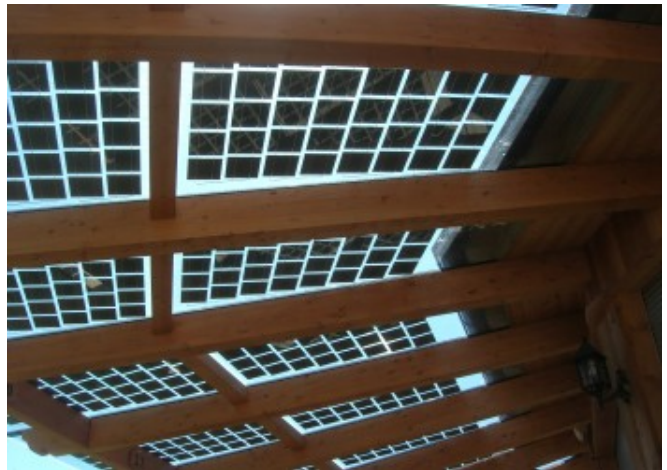
Timber structure hiding the modules fixing system © Augustin Clement
