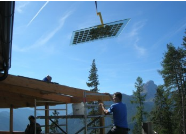
Construction phase, the frameless modules are easily mounted © Augustin Clement
