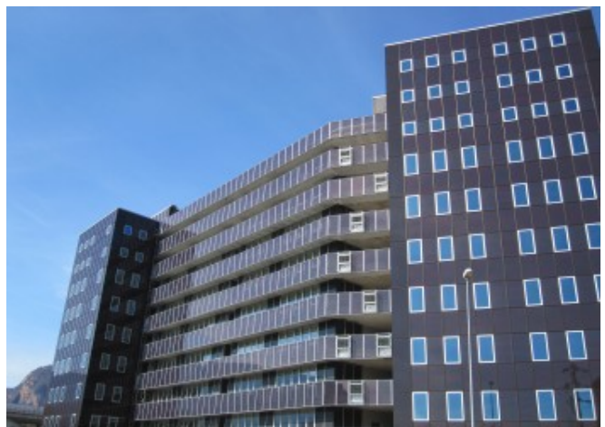
The building shows an impressive appearance highly visible from the surrounding areas © Eurac Research
