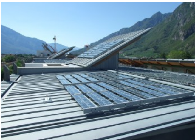
Glass-Tedlar modules (a) mounted on metal frames fixed to the buildings' roof © FAR System Srl
