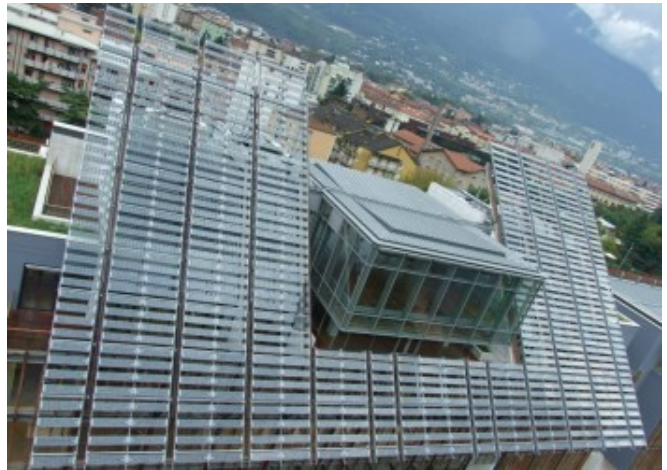
The BIPV system is highly visible as a key element in the whole building composition © FAR System Srl
