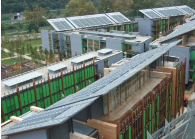
The modules are placed on the most of the district buildings as a unifying element © FAR System Srl
