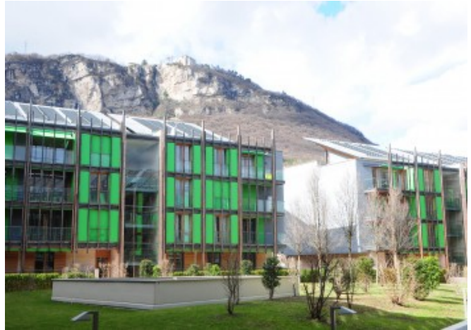
The buildings follow the surrounding mountain environment with different heights and inclinations © Eurac Research
