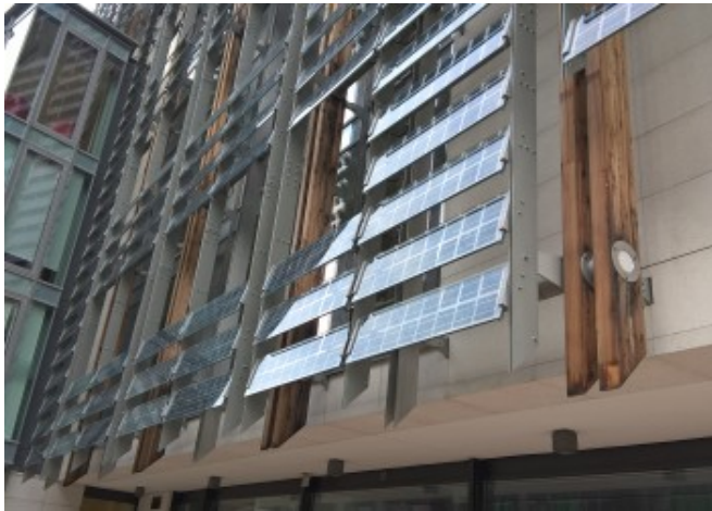
Glass-glass modules (b) anchored with special clamps to existing structures © FAR System Srl
