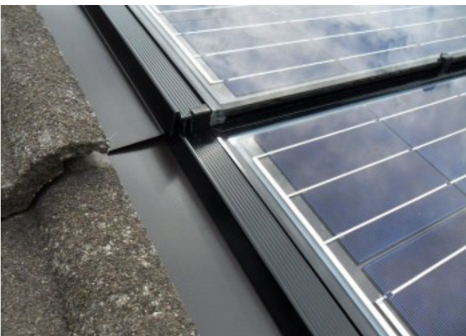
Detailed view of the 'Solrif' mounting system © Ing. Studio Blasbichler Srl
