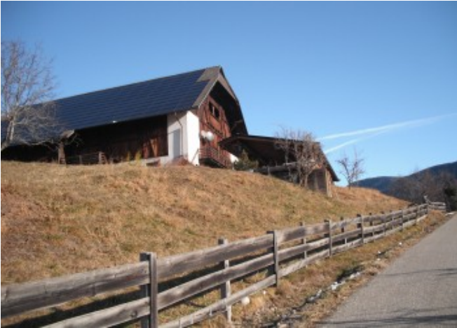
The building embedded in the mountain surrounding of the Salto high plateau © Ing. Studio Blasbichler Srl
