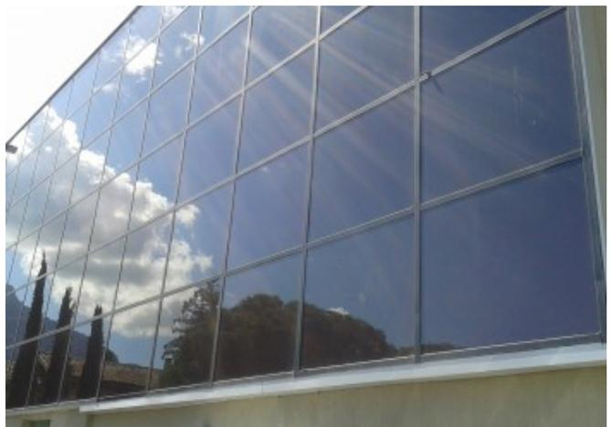
The thin-film modules create a high aesthetic quality building façade with a homogenized surface © Eurac Research
