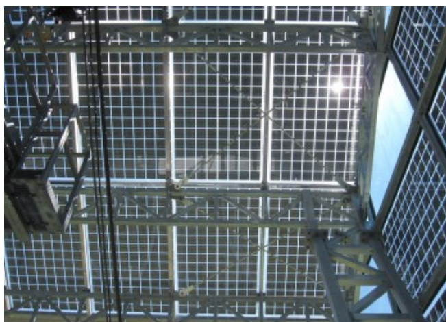
Detailed view of the glass modules mounting structure © Leitner Electro Srl
