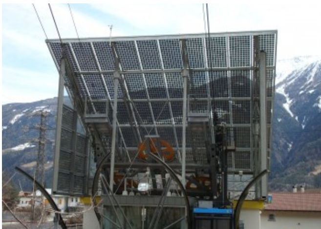
View of the downstream unit semi-transparent glass roof © Eurac Research
