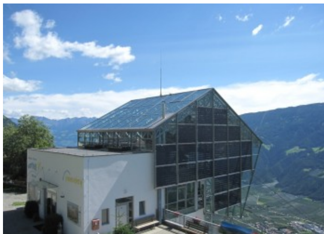
View of the upstream unit semi-transparent glass façade © Leitner Electro Srl
