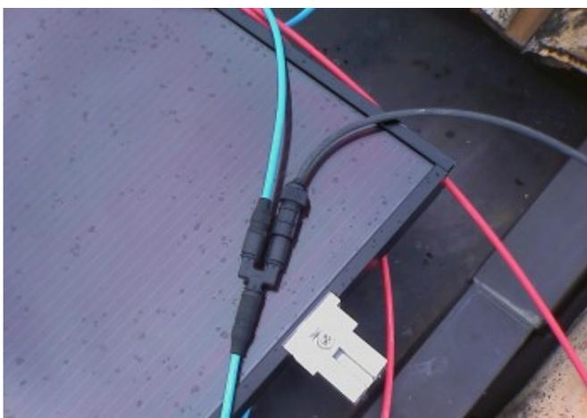
Detailed view of the modules cables and the special fixing grab © building owner
