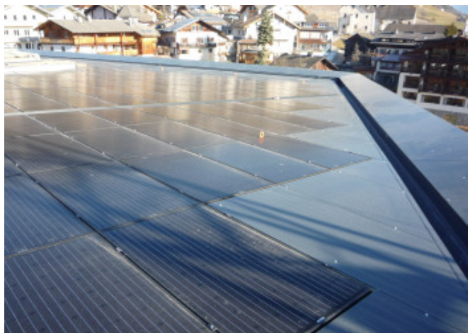
Final modules are installed, finishing the BIPV plant surface © Arch. Albert Colz
