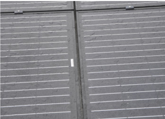
Detailed view of the modules © Elektrostudio
