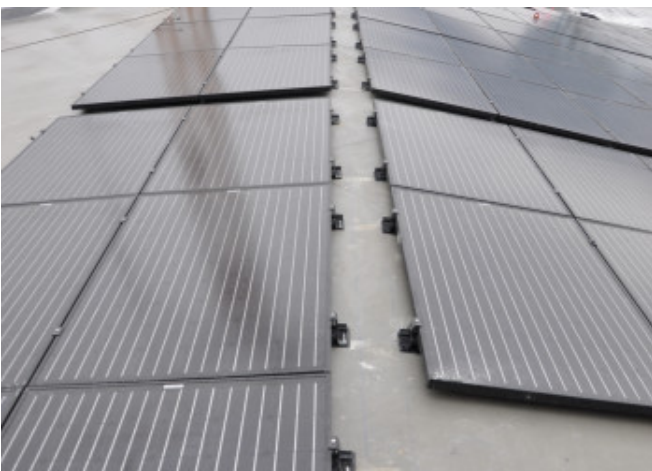
Space between the modules is left in order to permit through passage for the maintenance operations © Elektrostudio
