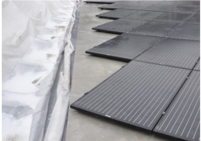
The innovative BIPV technology is used within a traditional urban context © Elektrostudio
