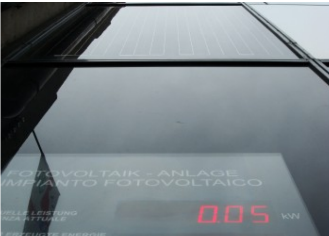
The photovoltaic energy output is visible on the façade surface © Eurac Research
