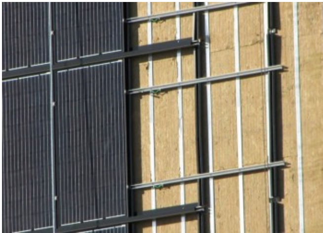
Mounting detail showing vertical Z-girts © Gordon Howell (HME)
