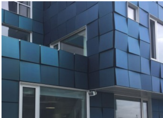
Detail of BIPV façade © Karin Kappel
