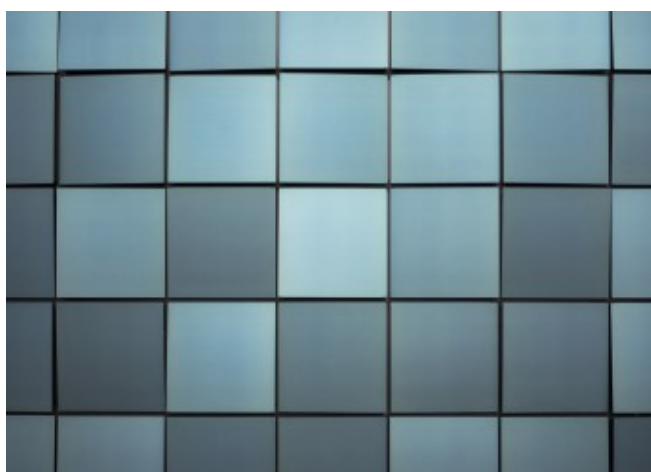
Close-up of the façade: the colours are depending on the angle of the module © C.F. Møller Architects / Adam Mørk
