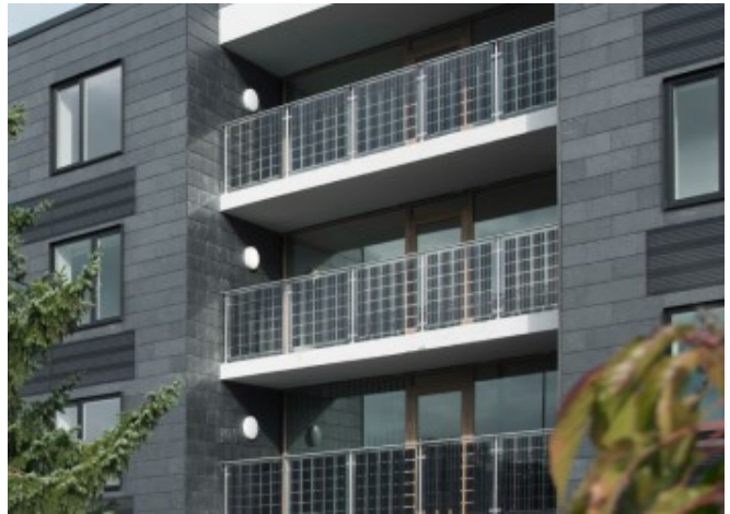
Semi-transparent BIPV modules in the balustrades © KANT Architecter
