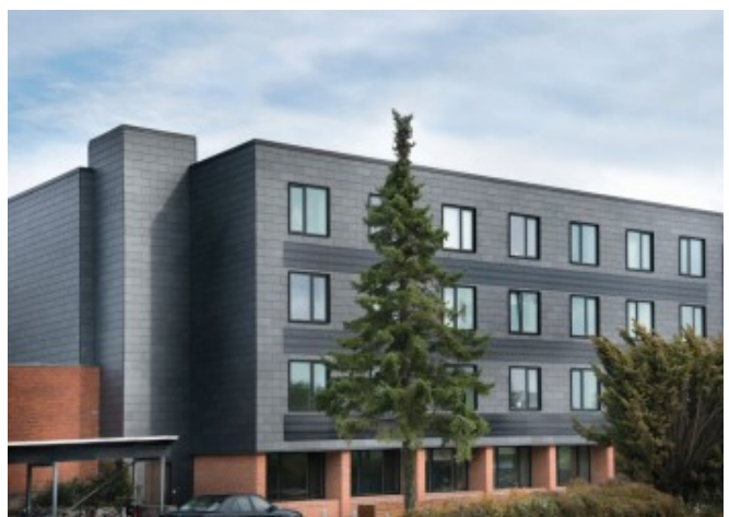
BIPV façade © KANT Architecter
