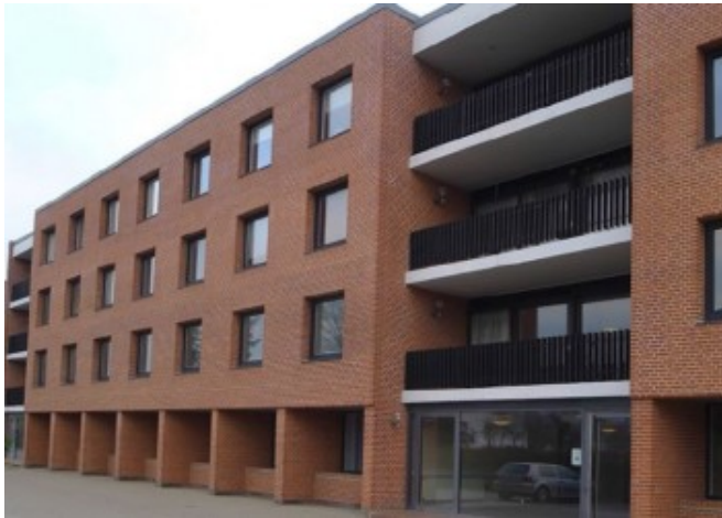
Apartments before the renovation © KANT Architecter
