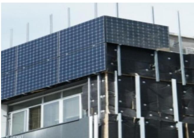
Renovation work details. PV modules mounting © CIEMAT
