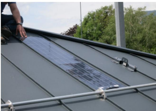
A Solbian photovoltaic module integrated into the roof © Arch. Valentina Cari
