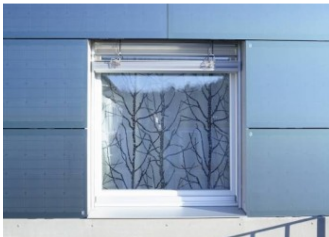
Detail of blue BIPV modules © Martin Zeller
