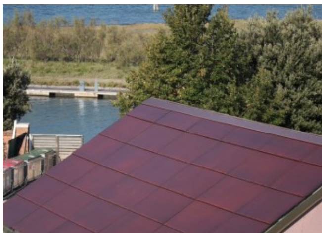
Building with photovoltaic tiles and the Venice lagoon in the background
