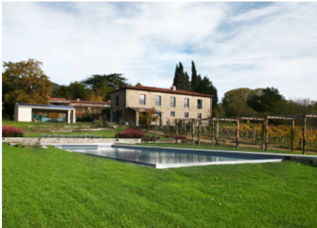
Technological pavilion with a BIPV roof annexed to the original twentieth-century building © Francesco Ferretti
