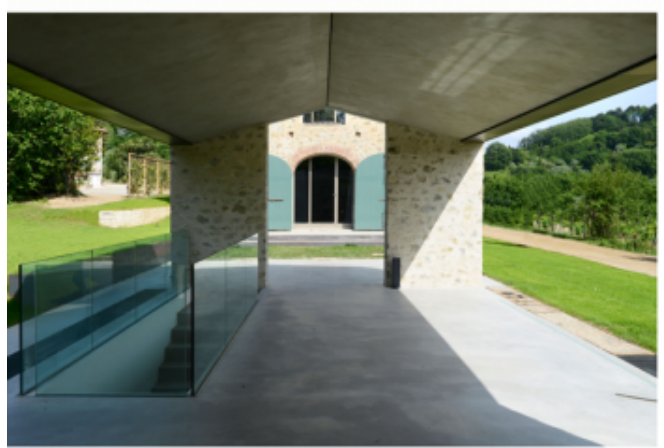
Relationship between the technological pavilion and the original main building © Beatrice Speranza
