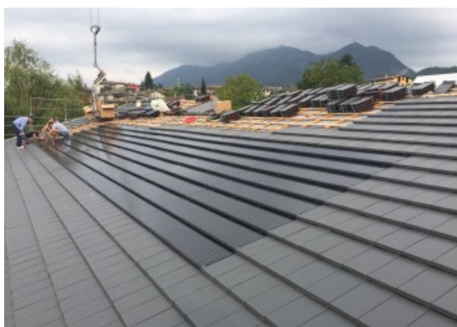
Positioning of tiles around the BIPV portion © marco minelli architetto
