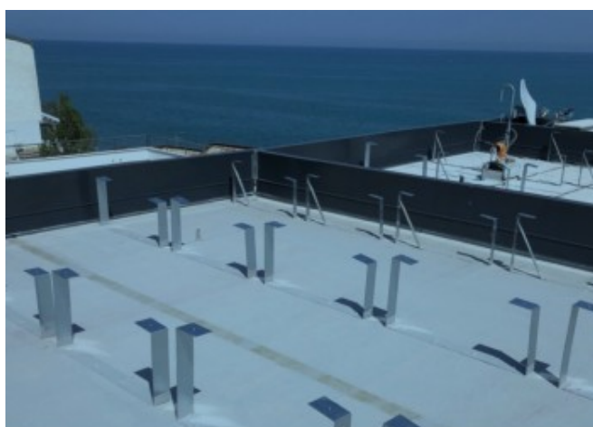
System for anchoring the modules to the canopy © Noemi Fabiano
