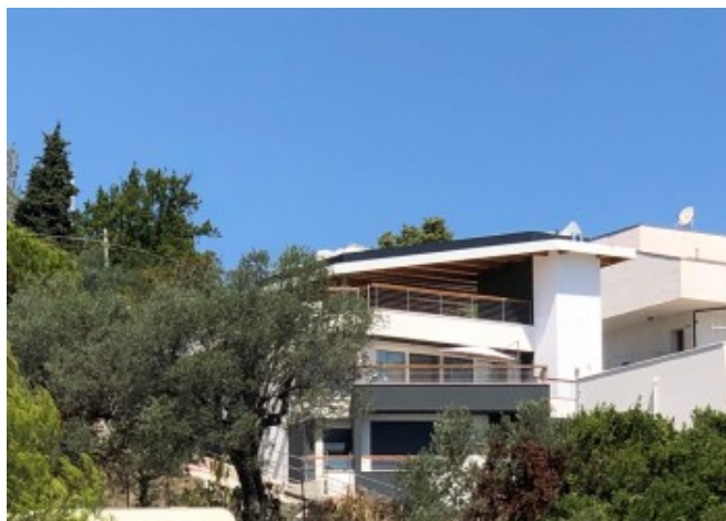
Close-up of the building in which the BIPV modules are not visible © Noemi Fabiano
